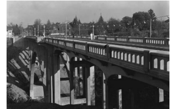
McKinley Elementary School building (above) and East 34th St Bridge in 1936. Source: Northwest Room at The Tacoma Public Library, Richards Studio T126-3 (bottom)
